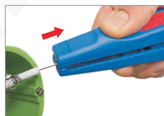
Stripping internal insulation
